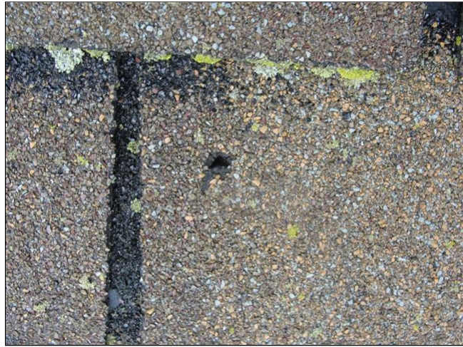
Holes in shingles / damaged shingles
