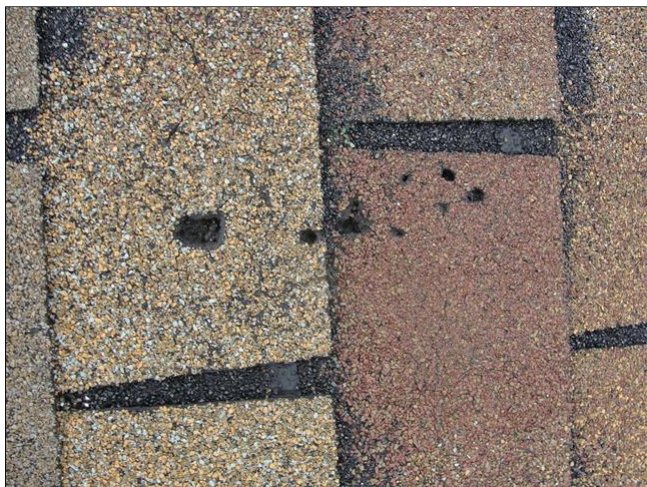
Holes in shingles / damaged shingles
