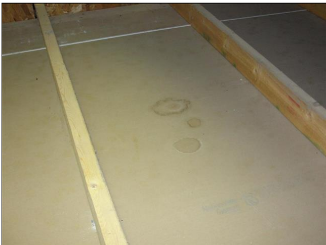
Stains below holes on garage ceiling
