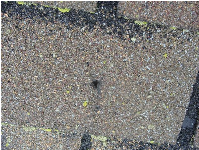
Holes in shingles / damaged shingles
