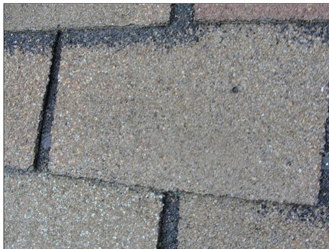
Holes in shingles / damaged shingles
