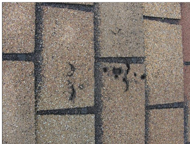
Holes in shingles / damaged shingles
