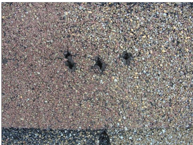
Holes in shingles / damaged shingles
