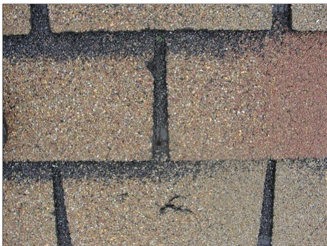
Holes in shingles / damaged shingles
