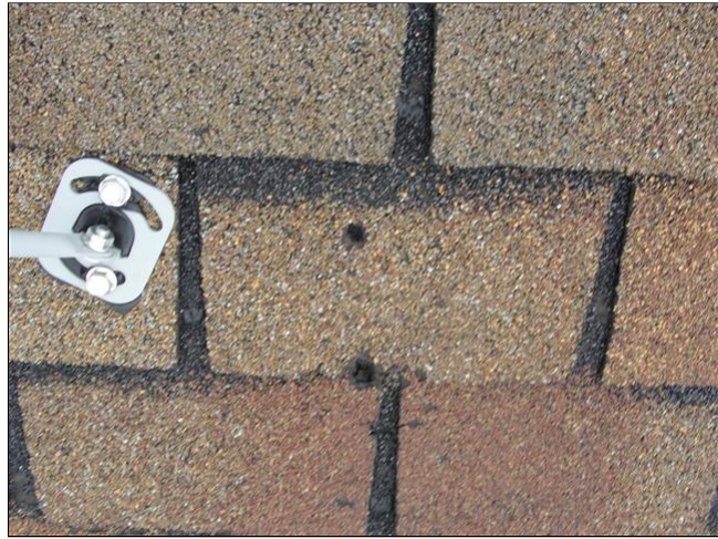
Holes in shingles / damaged shingles
