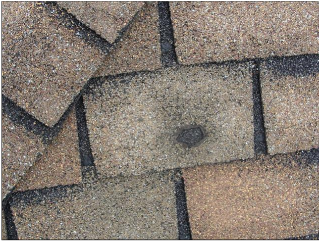
Holes in shingles / damaged shingles
