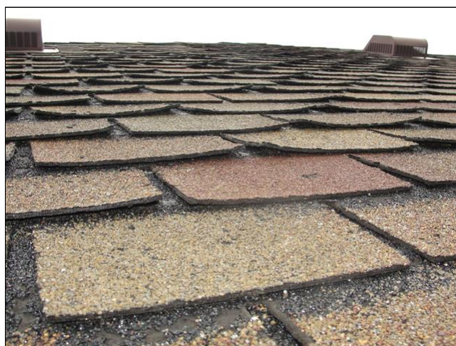
Deteriorated shingles
