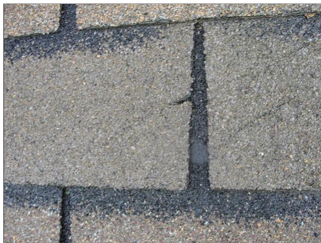
Holes in shingles / damaged shingles
