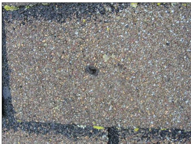
Holes in shingles / damaged shingles
