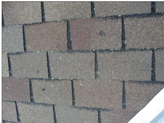
Holes in shingles / damaged shingles
