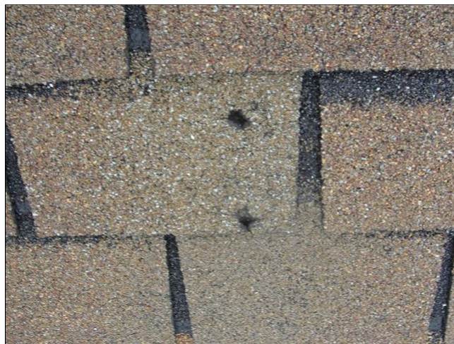
Holes in shingles / damaged shingles
