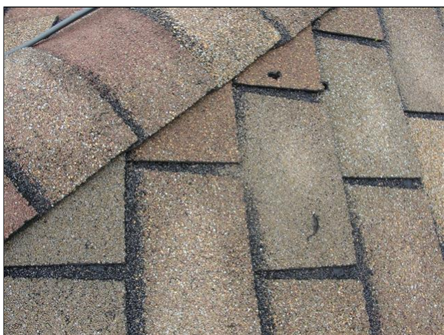
Holes in shingles / damaged shingles
