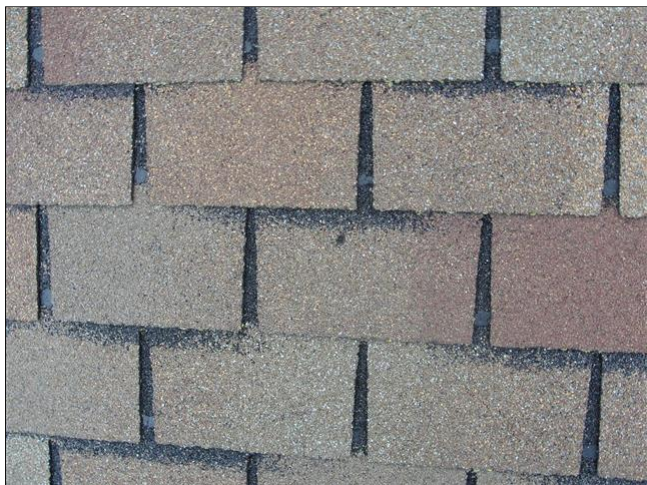
Holes in shingles / damaged shingles
