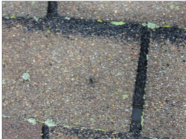
Holes in shingles / damaged shingles
