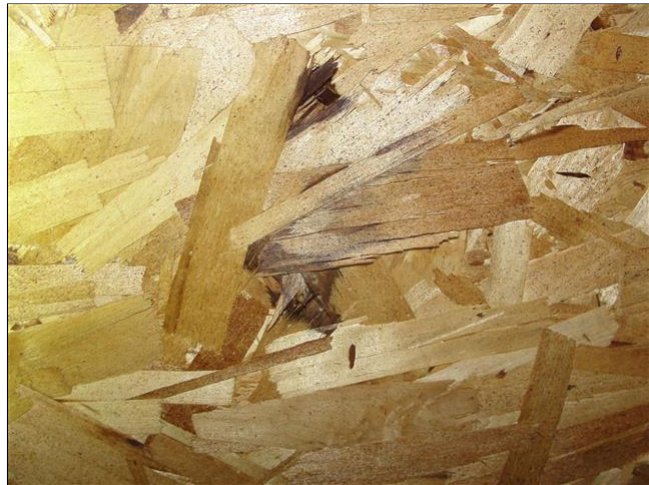
Stains on roof sheathing visible from garage attic
