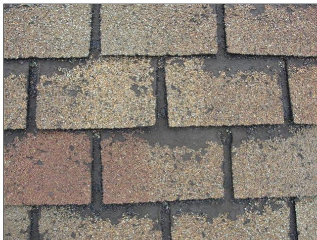
Deteriorated shingles
