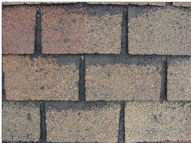
Deteriorated shingles
