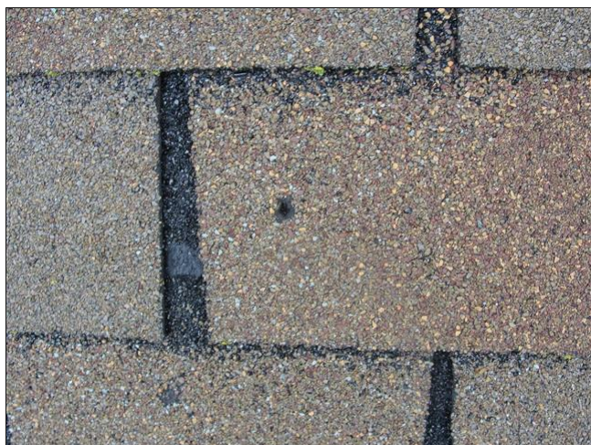
Holes in shingles / damaged shingles
