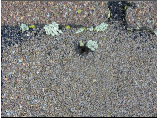
Holes in shingles / damaged shingles
