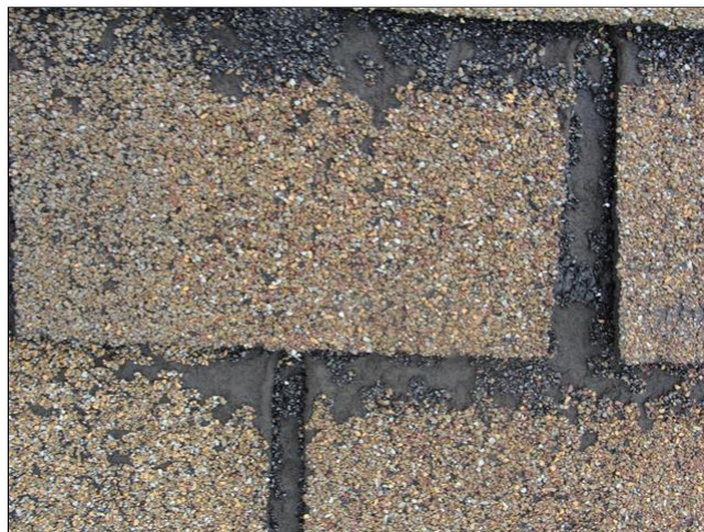
Deteriorated shingles
