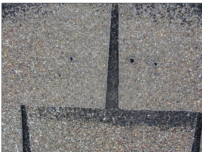
Holes in shingles / damaged shingles
