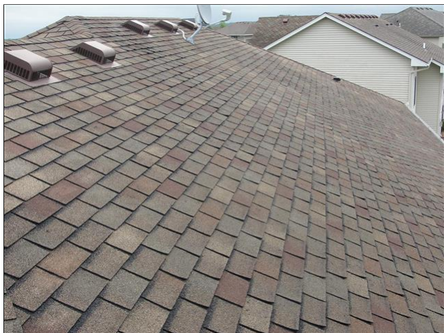
Deteriorated shingles
