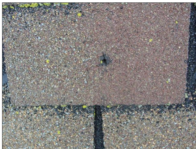
Holes in shingles / damaged shingles
