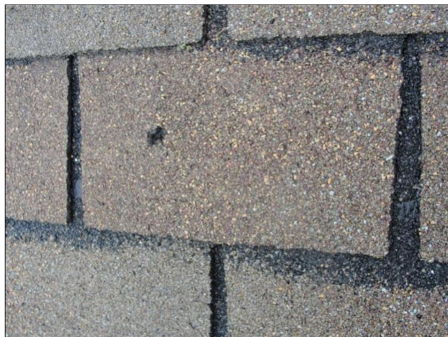
Holes in shingles / damaged shingles
