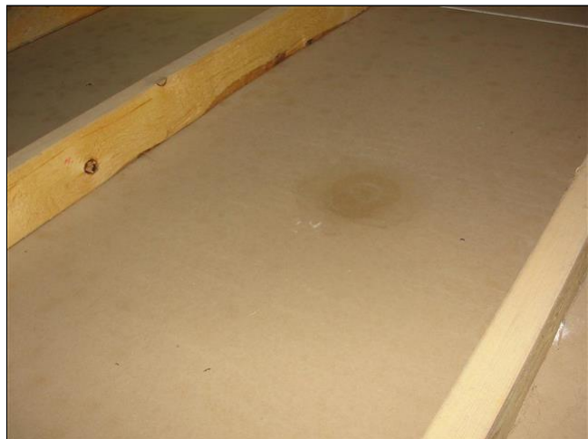
Stains below holes on garage ceiling
