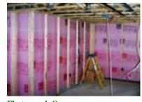
Photograph 8 Unfaced extruded polystyrene against basement wall
