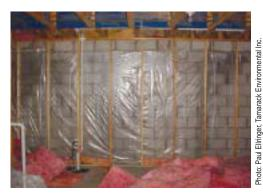
**Photograph 6**Water trapped behind polyethylene installed directly against foundation wall
