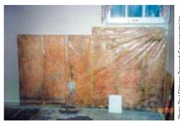
**Photograph 5**Frame wall with interior vapor barrier resulting in mold, decay and odors
