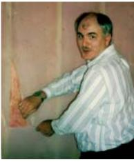
Photograph 2 Interior basement stud framing insulated with fiberglass batts and covered with a polyethylene vapor barrier
