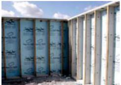
**Photograph 11**Pre-cast basement walls with XPS foam insulation
