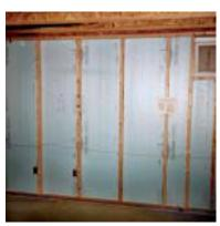
Photograph 9 Unfaced extruded polystyrene against basement wall
