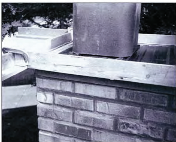
Crown and wash forms prepare a new chimney top.
