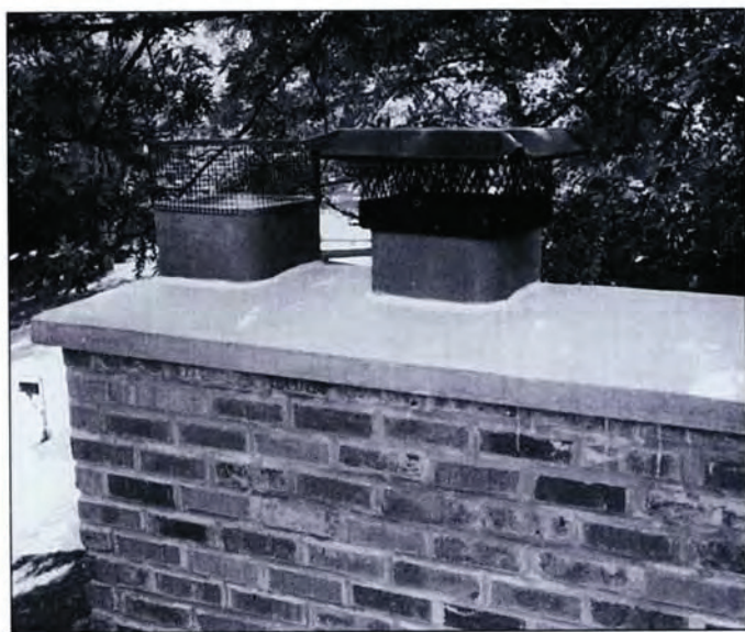
A freshly poured concrete crown is set to protect this masonry chimney for years to come.
